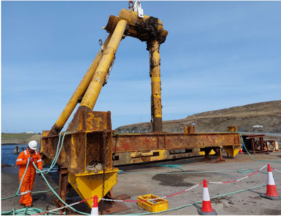
Figure 2: Inspection of 8-year-old substructure showed no notable deterioration
