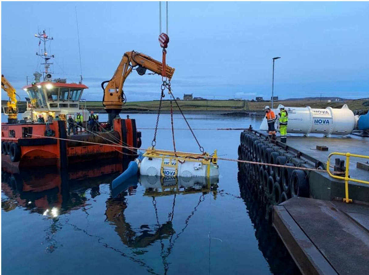
Figure 9-1: T5 and T6 turbine load-out (LARS frame in yellow)
