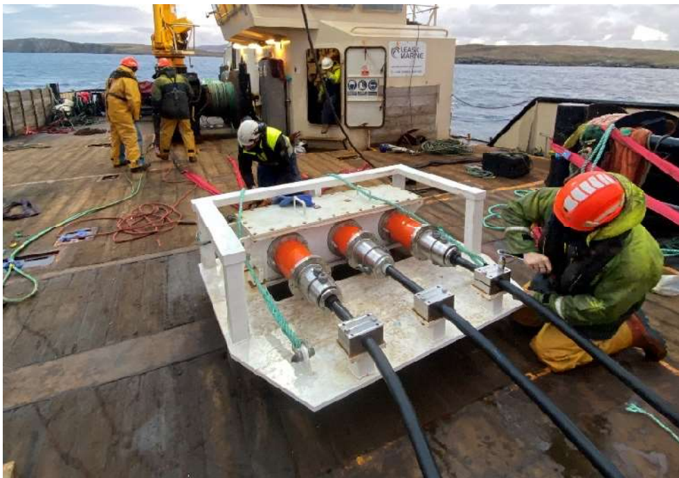
Figure 7: T5/T6 subsea cable hub on deck prior to installation
