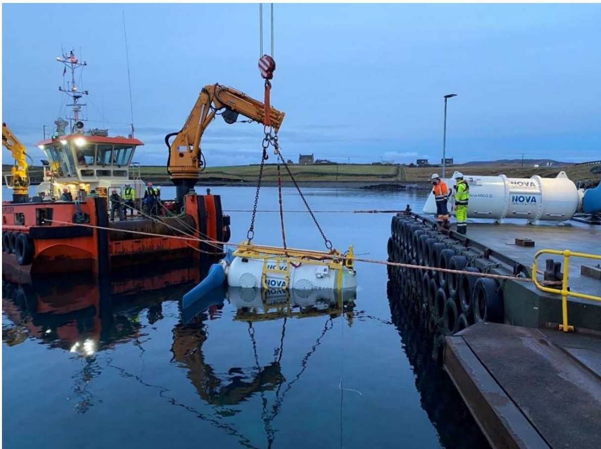
Figure 9: T5 and T6 turbine load-out (LARS frame in yellow)
