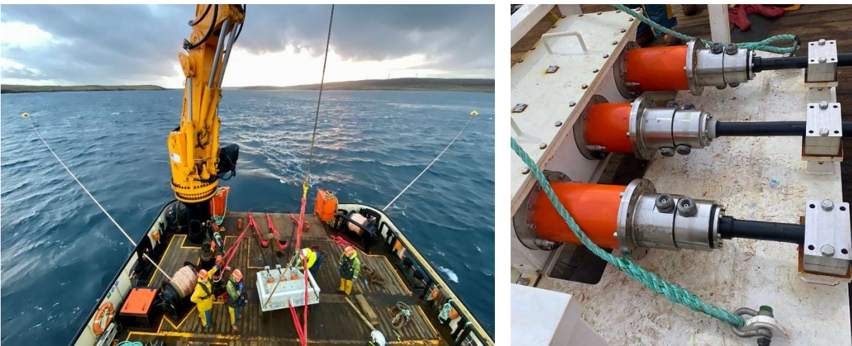
Figure 8: T5/T6 subsea cable hub installation
