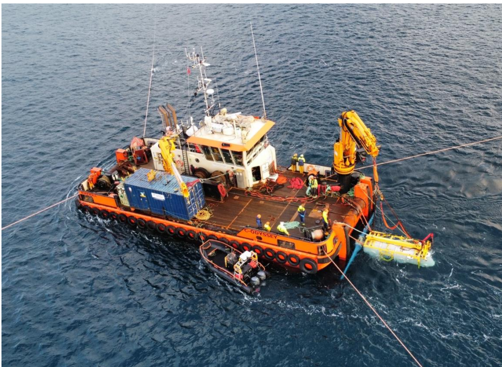
Figure 8: View of turbine deployment. LARS is yellow frame on top of turbine
