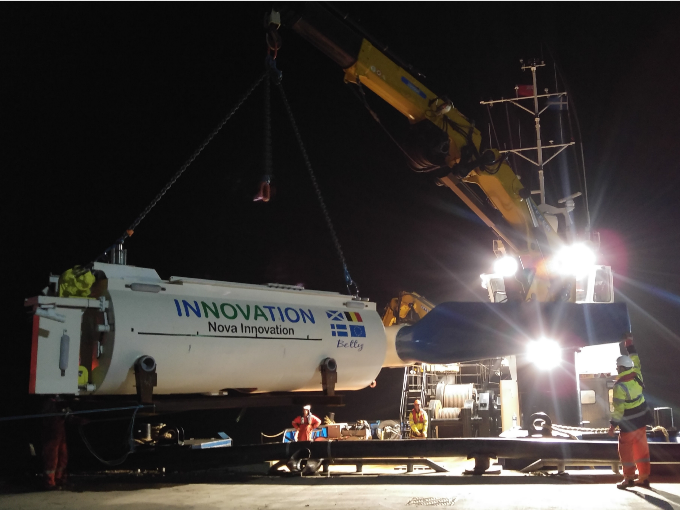
Nova Innovation M100 turbine being deployed in Shetland
